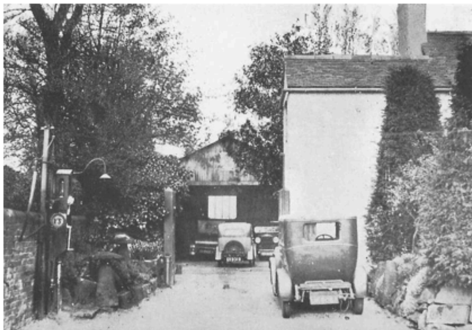
The former Harpers Garage in Wolverhampton Road, Codsall. (1935)
